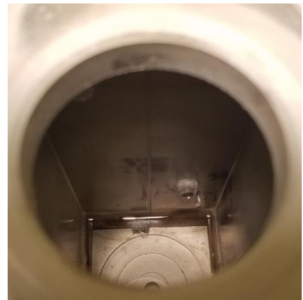
Reservoir B water level after leak.
