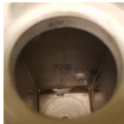
Reservoir B water level after leak.
